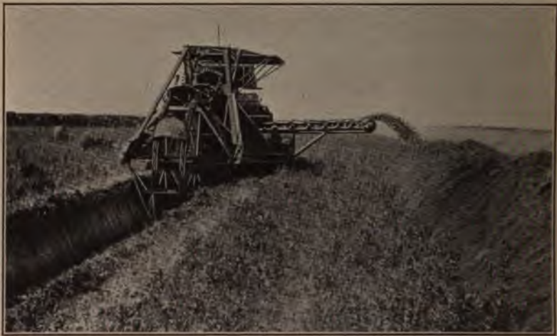
Wheel Excavator Constructing Small Ditch.
